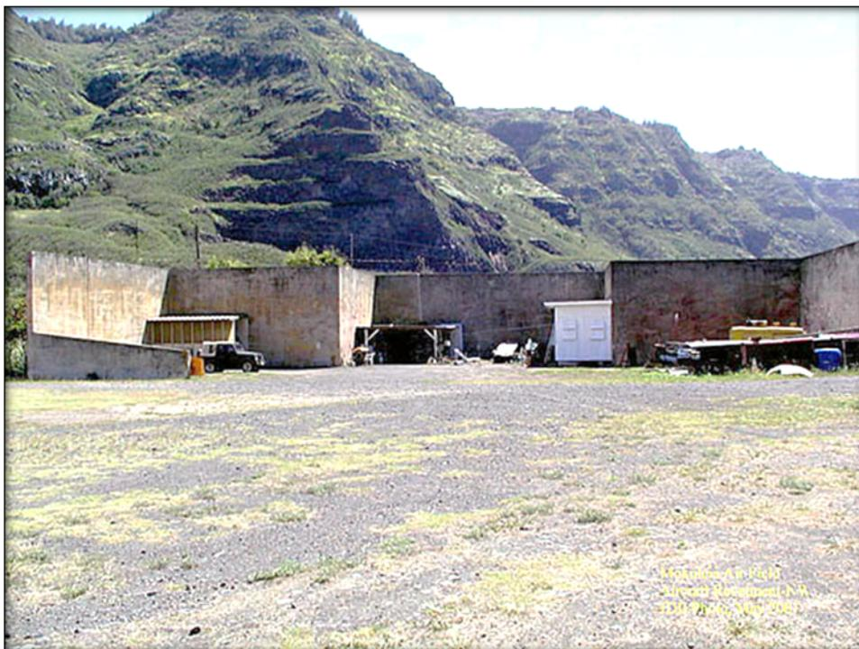
The above pictured revetment was built of reinforced concrete, one of two extant at Dillingham Airfield from WWII. Note the various compartments. (Photo by author)
