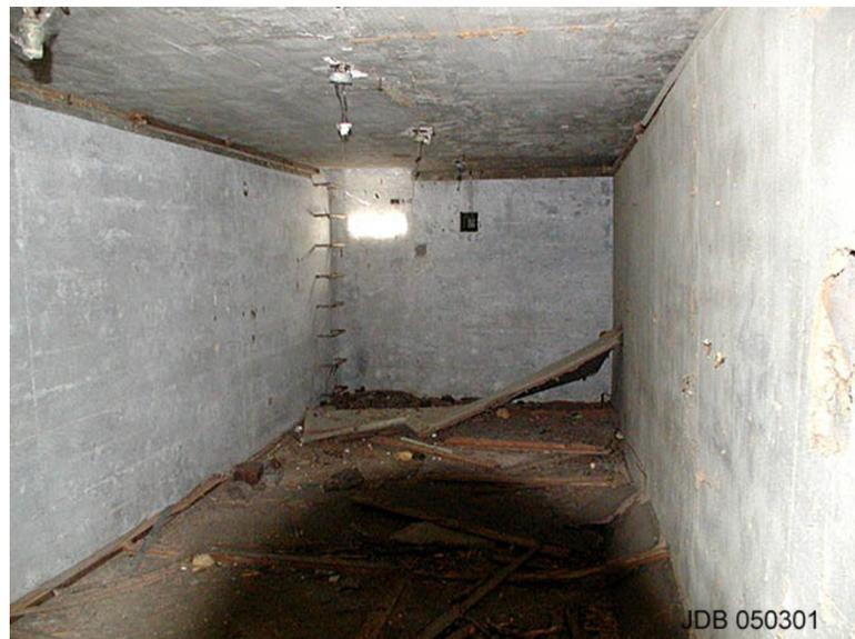
Interior of CP at Dillingham Airfield. Interior dimensions were: 21' 0" x 9'8" x 8'0" with walls approximately one foot thick. Note rebar rungs ascend to escape housing at the left rear. (Photo by author)
